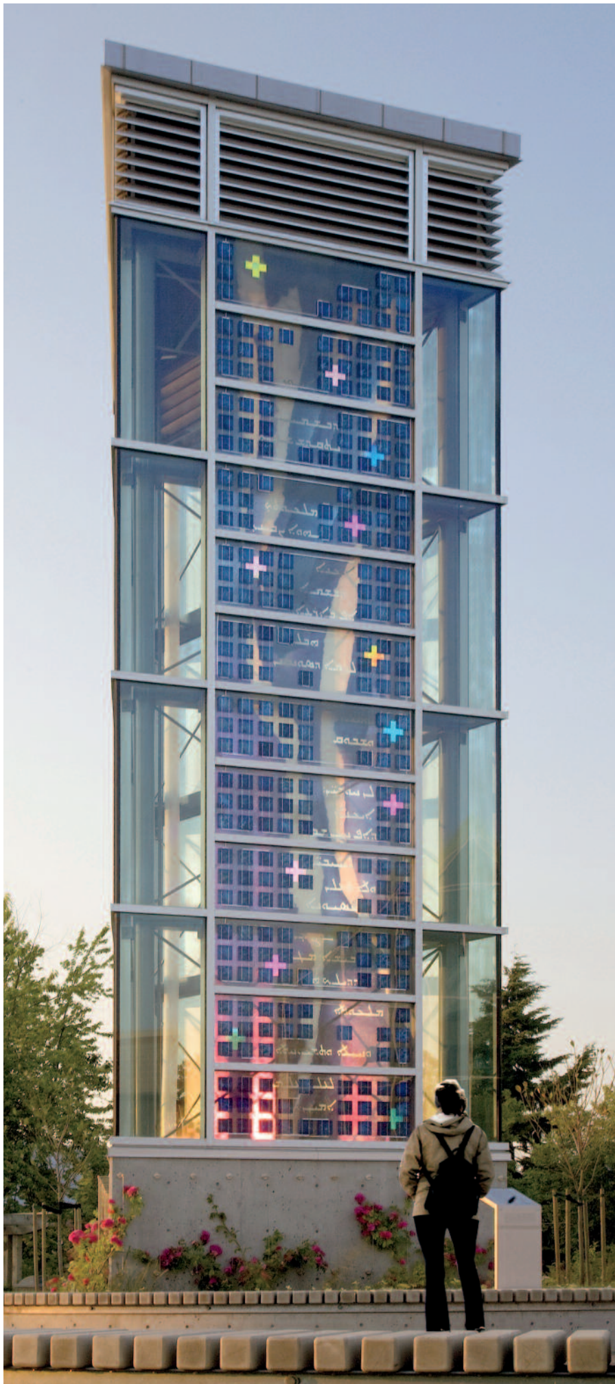
Lux Nova, daylight view of the wind tower, Regent College, Vancouver, BC ✦ 2007c
